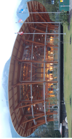
The 9,500 square foot Squamish Adventure and Visitor Info Centre, with its fir columns and eagle-wing roofing design elements, is a good example of how wood could be incorporated into the proposed Wood Showcase/Tourism Discovery Centre for Vancouver Island.
